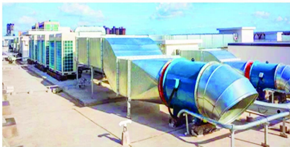
VRF ( Variable Refrigerant Flow )
